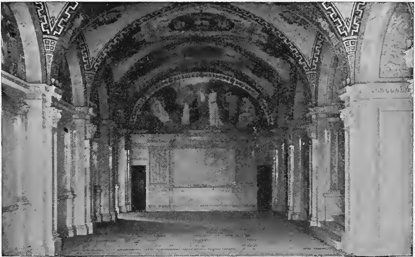
THE NORTH CORRIDOR. — MAIN ENTRANCE HALL.
